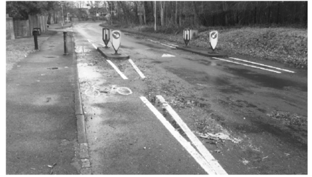
Cycle gap in horizontal deflection
